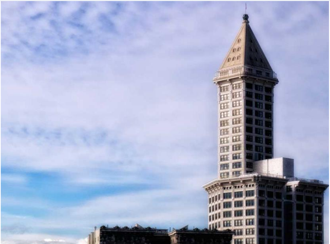
See all the way to the Seattle waterfront from the Smith Tower. Credit: David Lee
